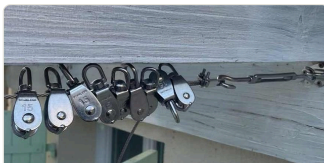
Tensioned cable with pulleys
