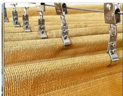
Rods clipped along the cable
